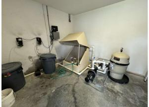
Pool equipment dates not provided. Pool filter and pump were recently replaced. Gas pool heater appears to be at the end of its useful life.
