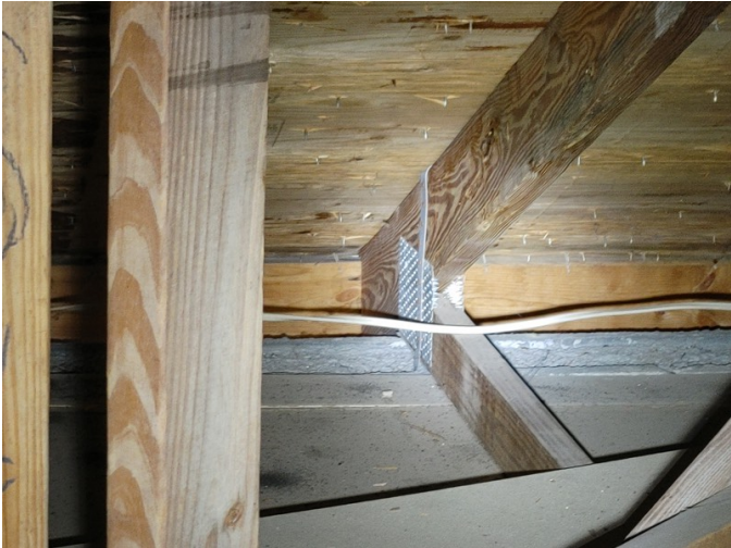
Wrap with 2 nails and 1 opposite side
