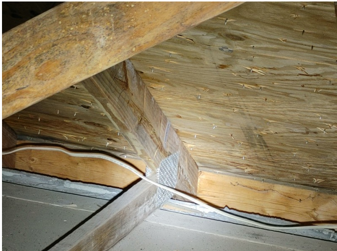
Wrap with 2 nails and 1 opposite side
