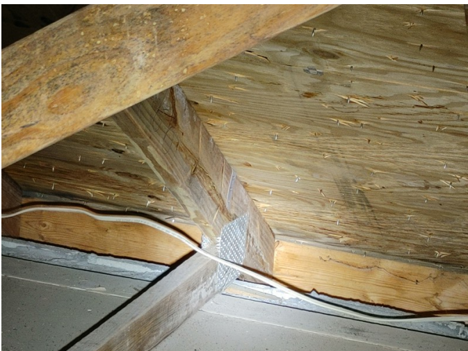
Wrap with 2 nails and 1 opposite side
