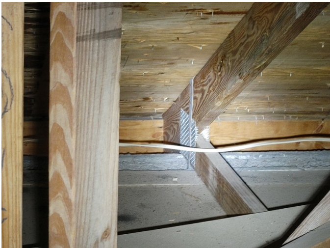
Wrap with 2 nails and 1 opposite side
