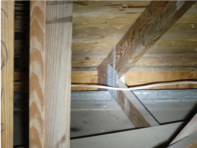
Wrap with 2 nails and 1 opposite side
