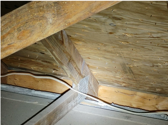
Wrap with 2 nails and 1 opposite side
