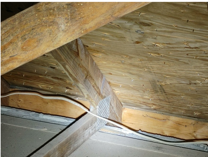
Wrap with 2 nails and 1 opposite side
