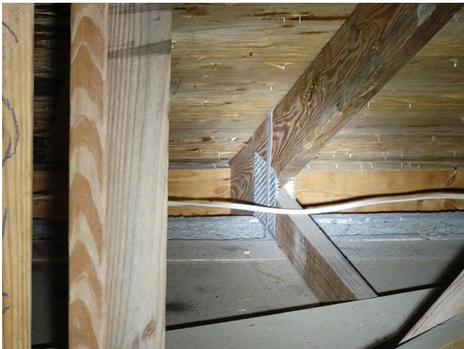
Wrap with 2 nails and 1 opposite side
