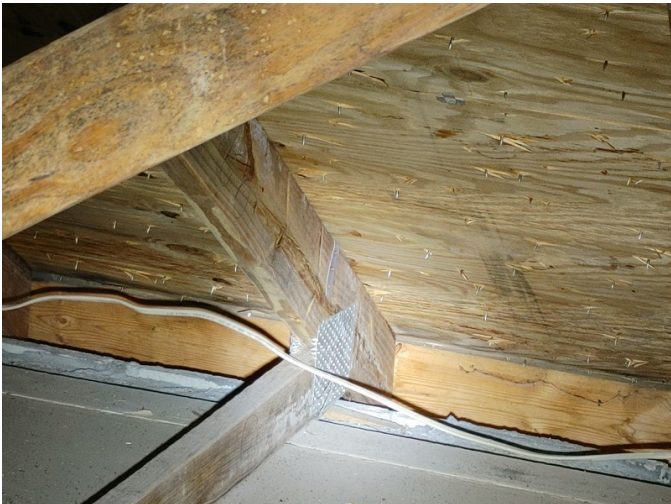
Wrap with 2 nails and 1 opposite side
