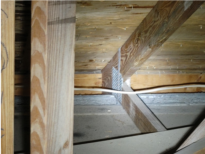
Wrap with 2 nails and 1 opposite side
